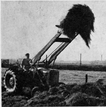
Front end loader, shown here with manure fork attachment
